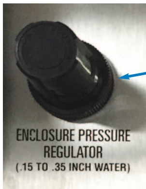
Figure F-14 Enclosure Pressure Regulator – Turn Clockwise
