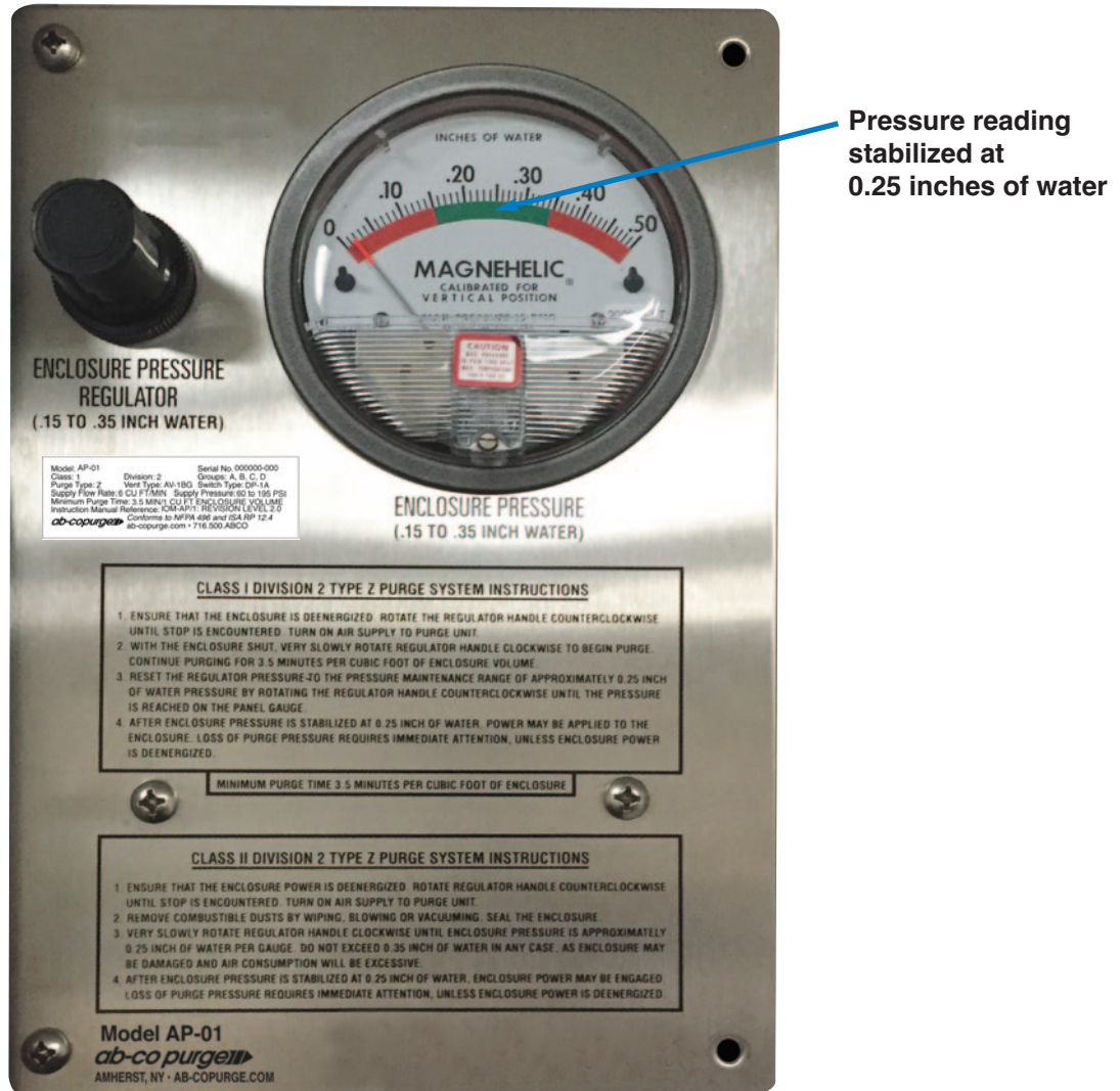
Figure F-16 AP-01 Front Panel (With Magnehelic Analog Gauge's Reading Stabilized at 0.25 inches of water)
