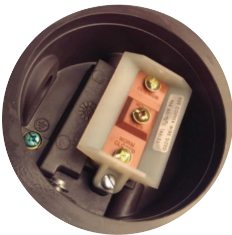
Figure R-5 DP-1A Terminal Block
